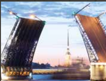
LIFT BRIDGE CONSTRUCTION
